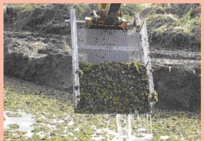
As the "Wire Mesh Basket" is lifted out of the ditch, the *Salvinia* plants are stuck on the screen for dumping.
