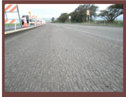
As previously stated, bonded concrete overlays can be placed on existing concrete, asphalt or composite pavements provided there is minimal structural damage. In regards to asphalt and composite pavements, the asphalt layer should not exhibit stripping or raveling or other materials-related issues.
