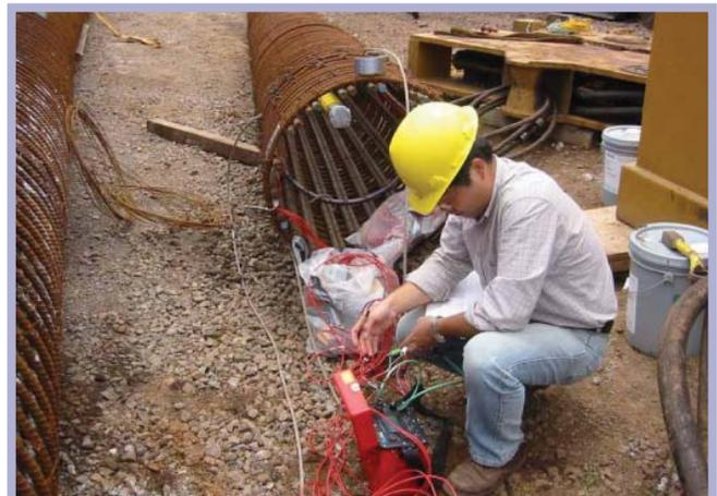
*Instrumented drilled shaft rebar cage with the inclinometer casing attached.*
