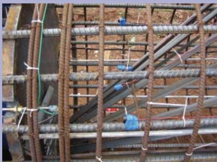
Trial shaft cage inner & outer log sensors.
