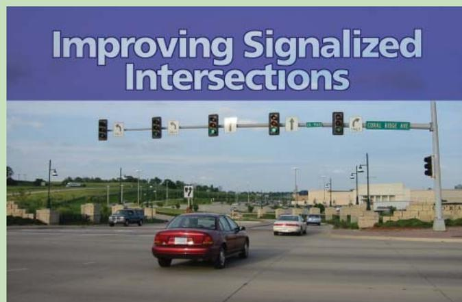
This intersection features lane-aligned signal heads (one signal head for each lane of traffic), with dual left-turn lanes, two through lanes, and a right-turn lane.
