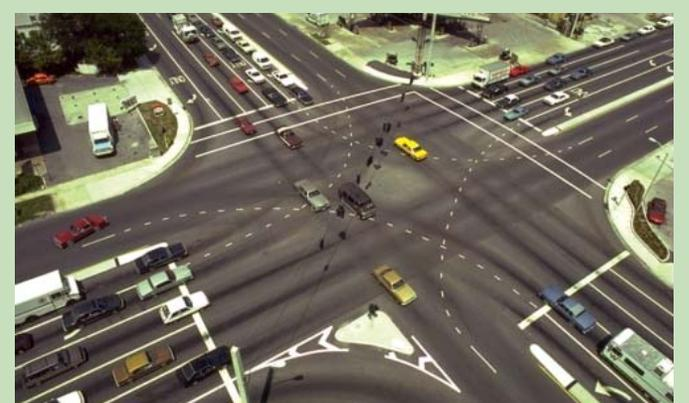
A well-designed signalized intersection can improve traffic safety and mobility. Pavement markings, like those shown in this overhead photo, can be used to delineate travel lanes within wide intersections.
