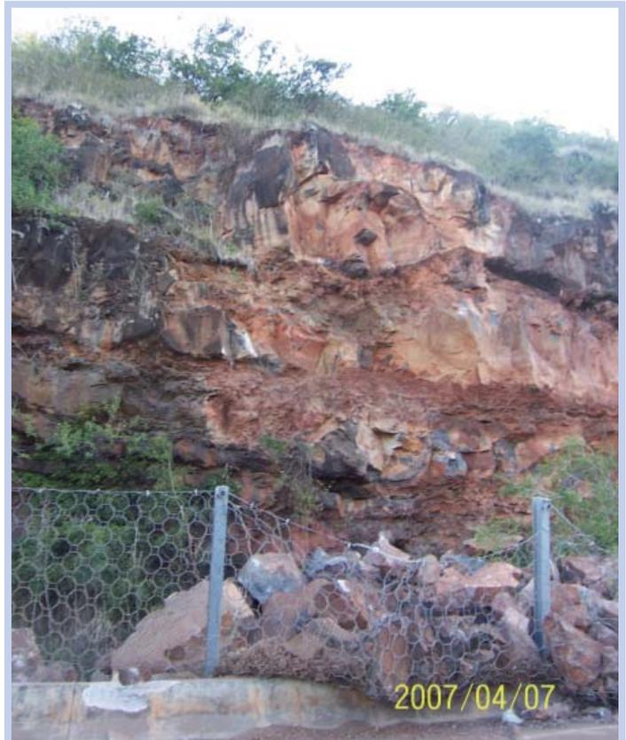
*Condition after April 2007 rockslide showing crushed rockfall fence.*
