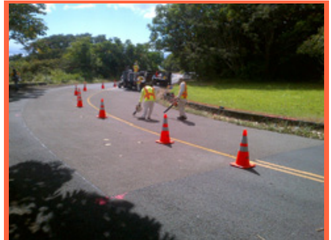
Construction on Tantalus Drive
