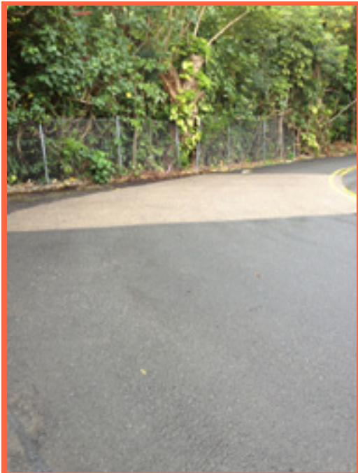
An installed “Tyre Grip”
