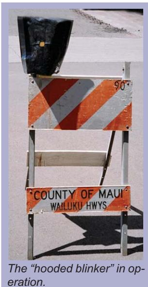
*The "hooded blinker" in operation.*
