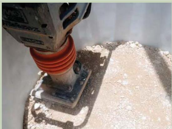
Fig. 1a: Compaction of coarse aggregate
