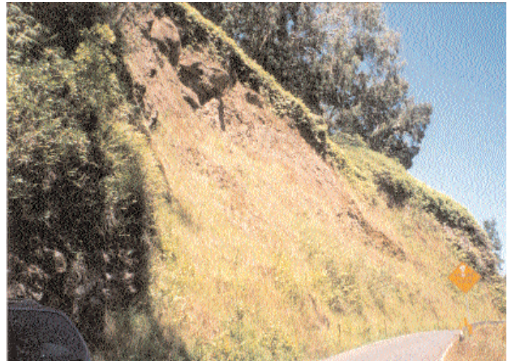
Above: Rock Slope along Hana Highway, M.P. 11.4 +/-, Maui.
